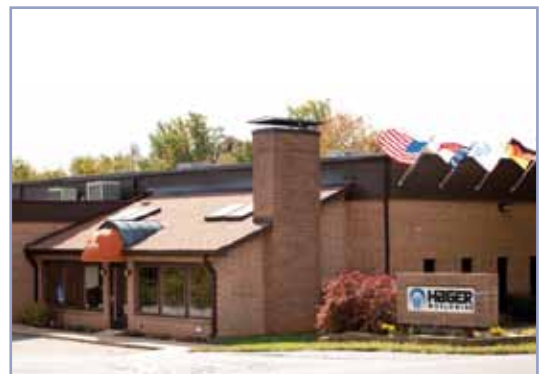
Hager Worldwide Corporate Office Hickory, North Carolina
