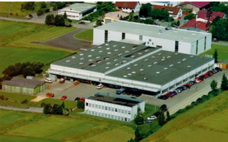
offices and factory in Langenau
